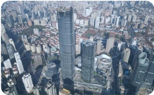
ITC·主楼 ITC Main Tower
